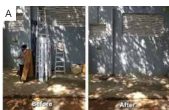
Location: Outside of the HT DG Control Panel Room
